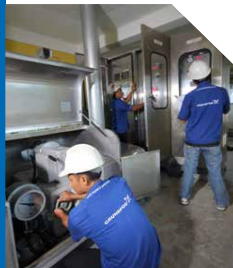
Grundfos Engineers supervise the installation.
